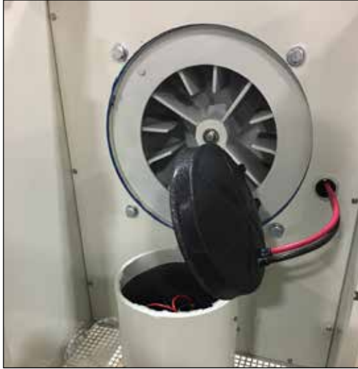
Figure 19 Installing the New Black Cover
