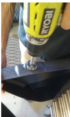
Figure 1 Drill hole in door panel
